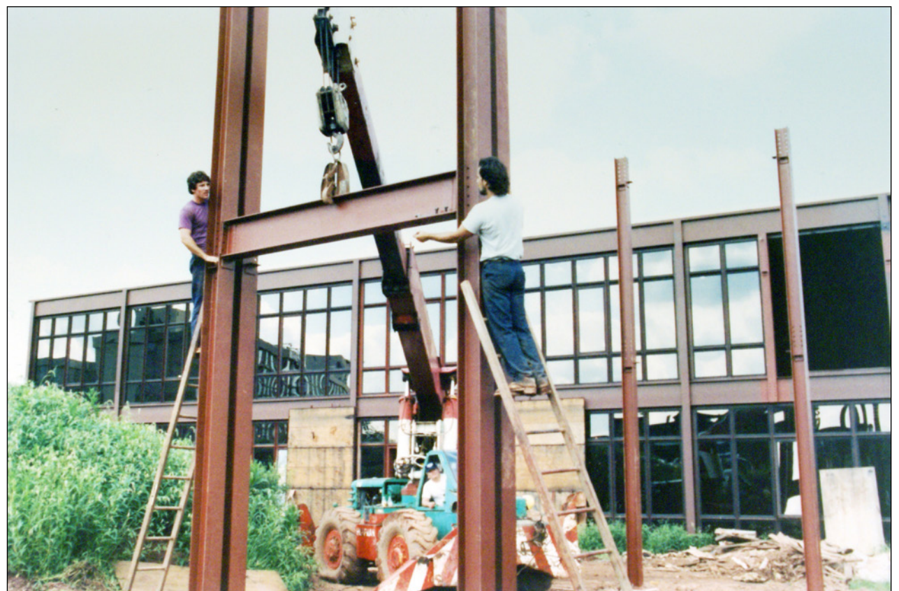
Bobby Pormili and John Zuchs work on supports for a bridge that will connect the first floor of the original building with the second floor of the one shown in the background.
