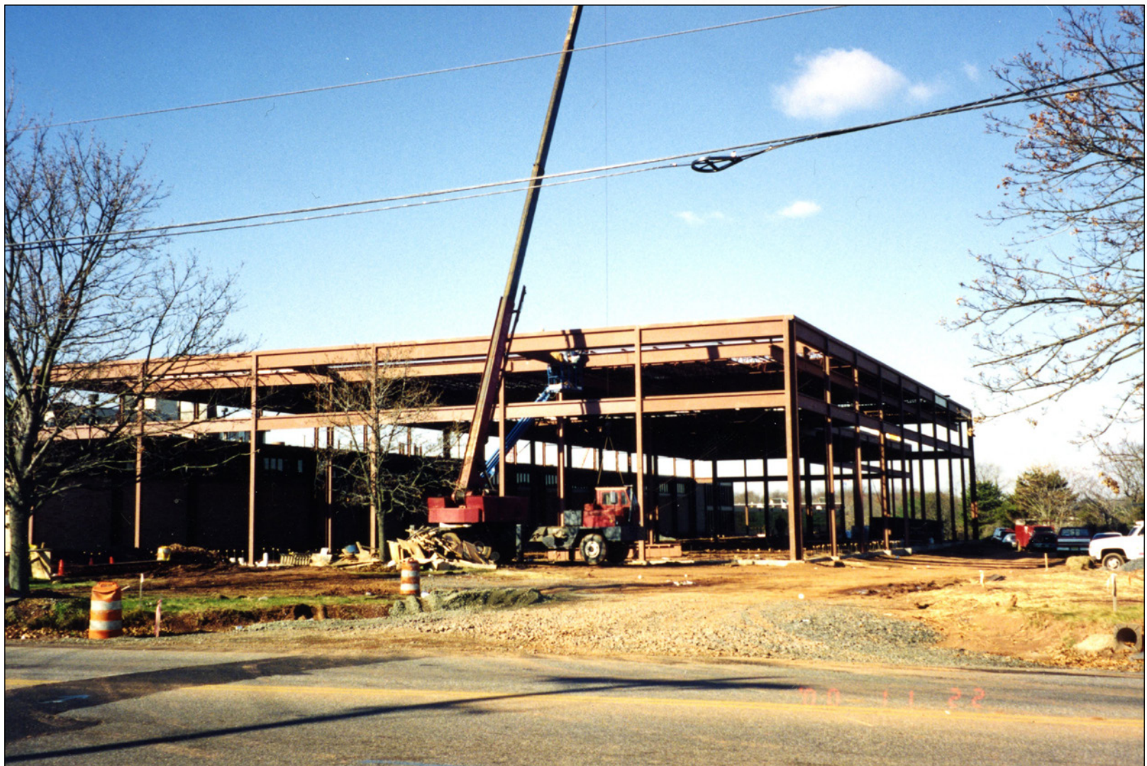
Building 1 A under construction. The view is from the front of the building on Davidson Avenue. (2000).
