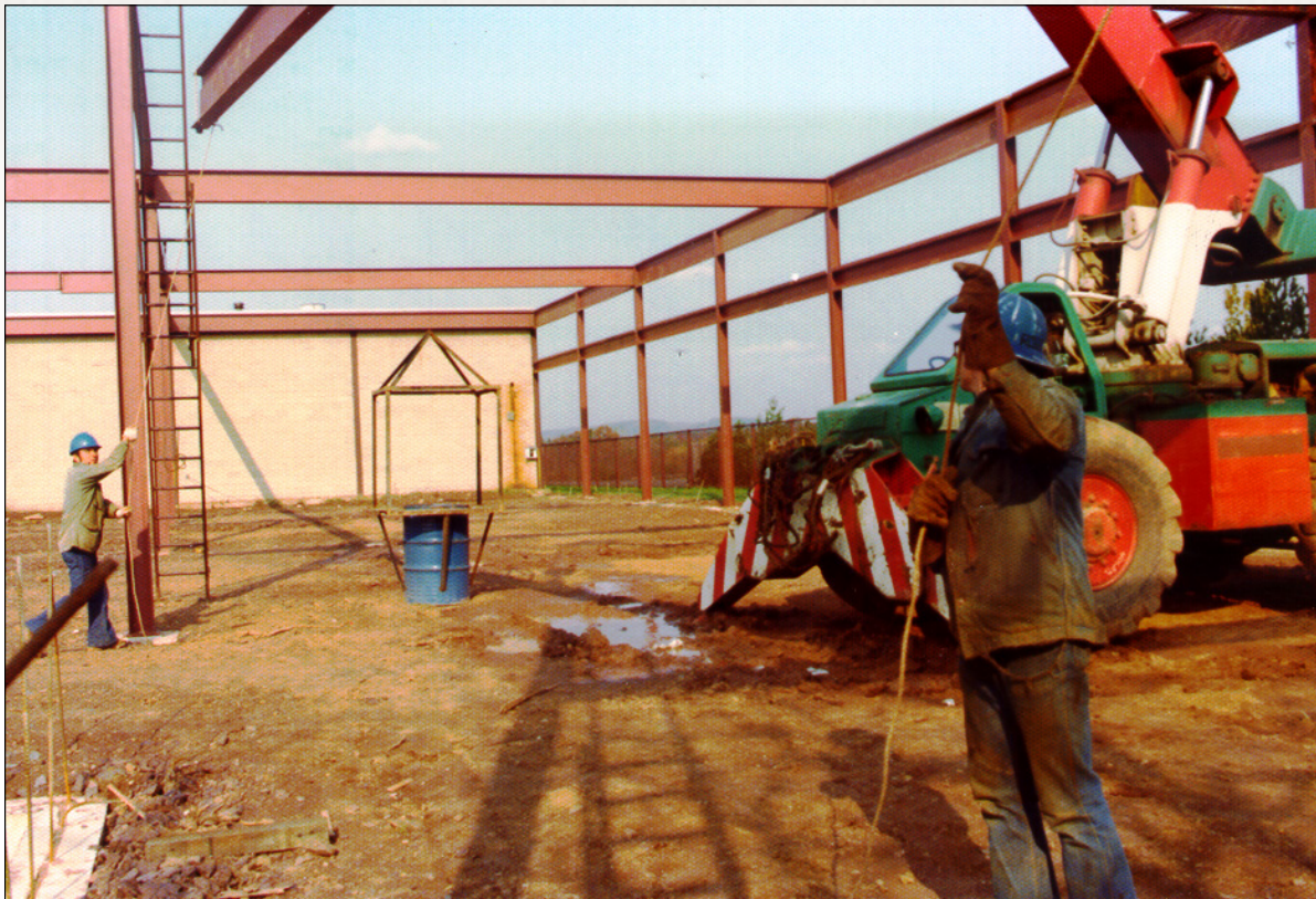
The crew joins one of several steel I-beams used in the construction of the first Rotor Clip building in 1971.
