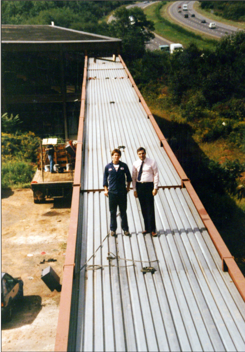
Craig Slass (left) and Joe Cappello survey the work on the bridge connecting Buildings 1 and 2.
