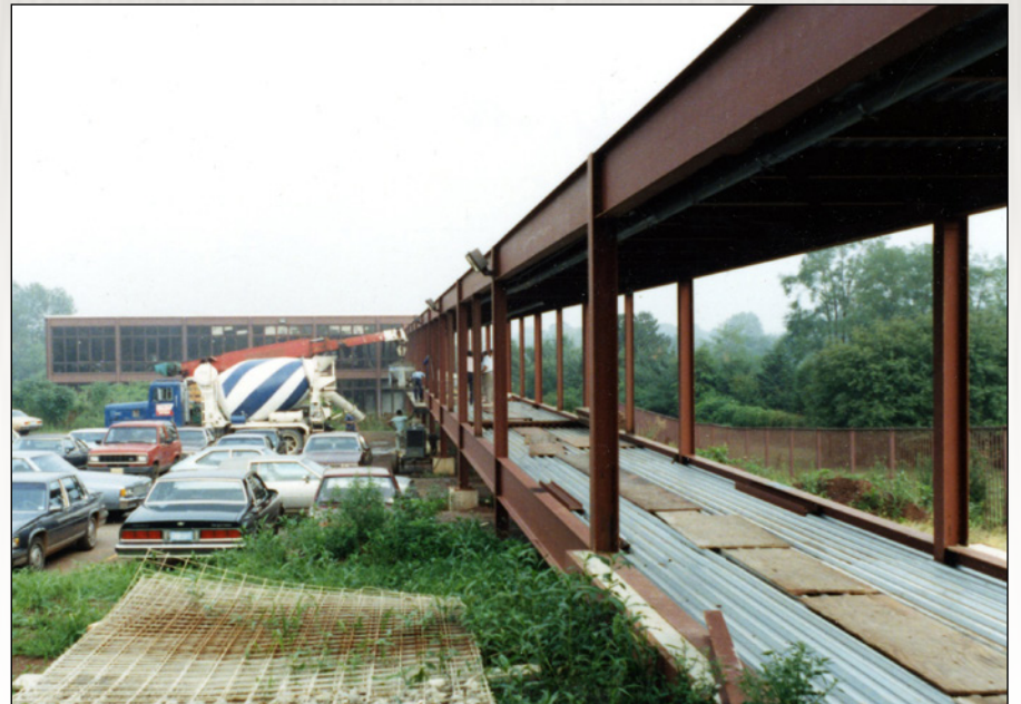
View from Building 1 showing bridge connecting the first floor with the second floor of Building 2
