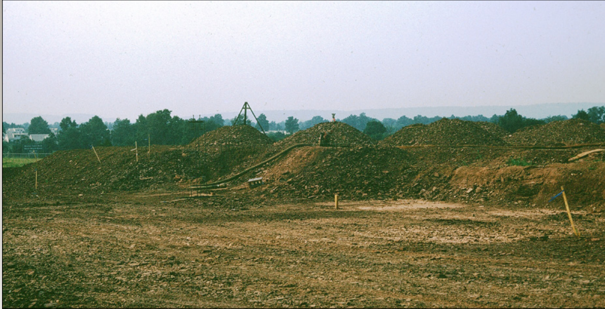
The land for the building was a parcel of former farmland in Central New Jersey. It bordered the then new Route 287, which would become a popular truck shipping route for Rotor Clip products.
