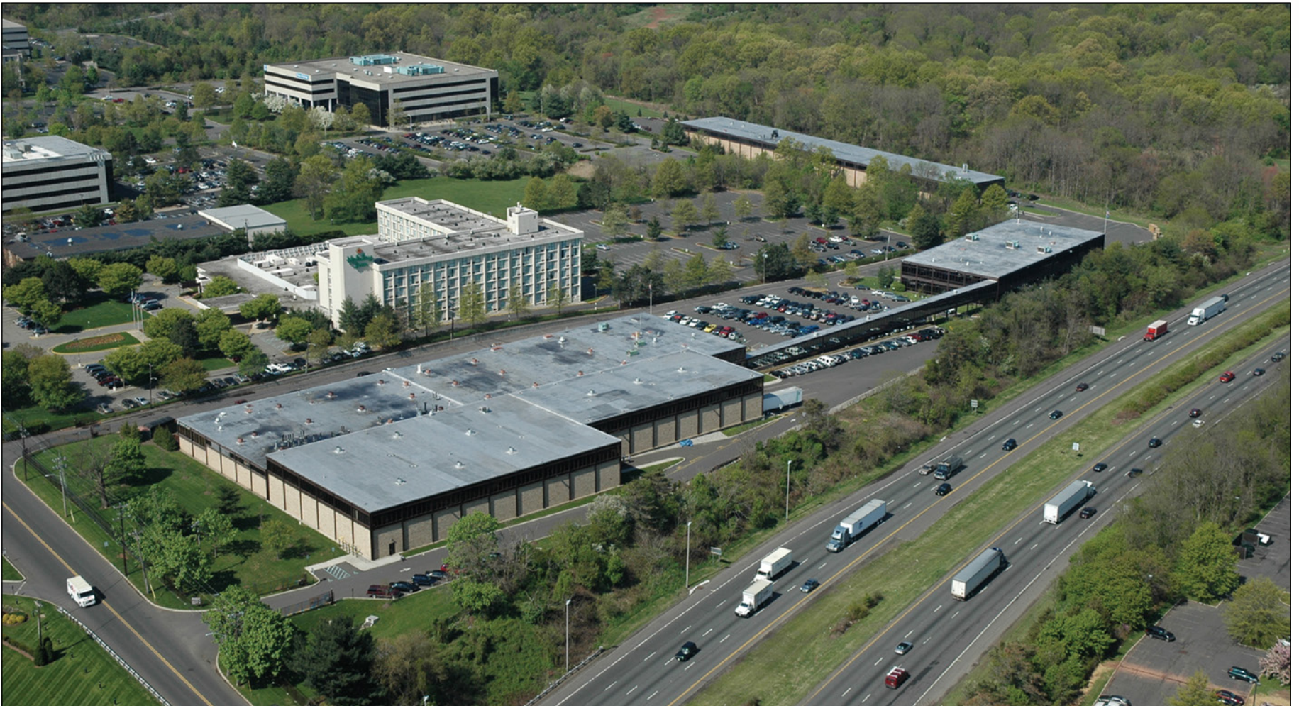
An aerial view of Rotor Clip USA showing Buildings 1, 2 and 3.
